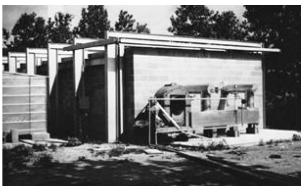
FIGURE A.38.3.2(b) View of Firing Mechanism of Fire Test Building.
