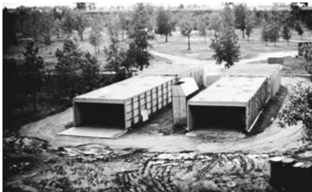
FIGURE A.38.3.2(a) Overall View of 20 ft × 100 ft (6.1 m × 30.5 m) Fire Test Building from Exhaust End.
